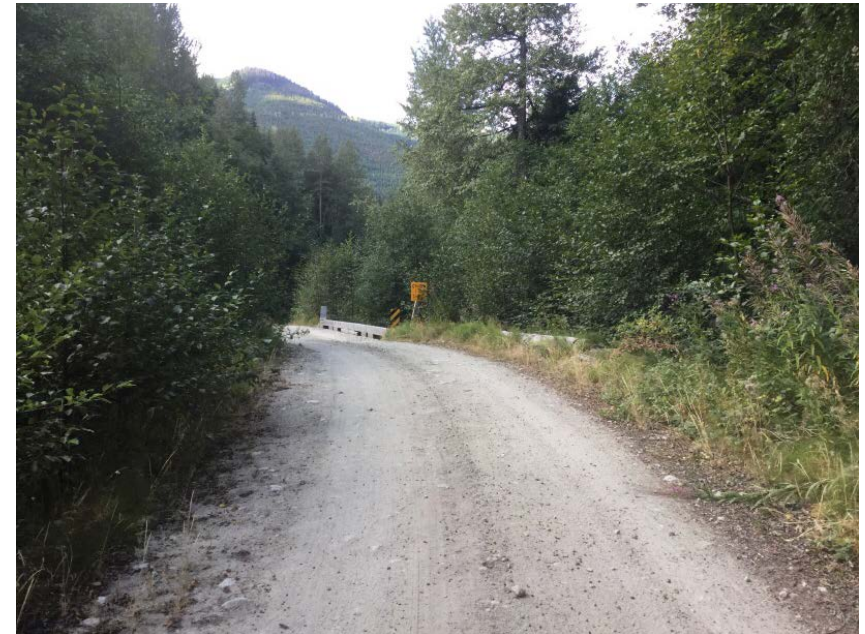
Approach from Right Bank when facing downstream
