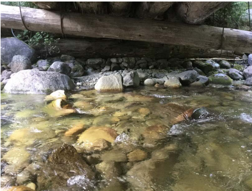
Left Bank Abutment when facing downstream
