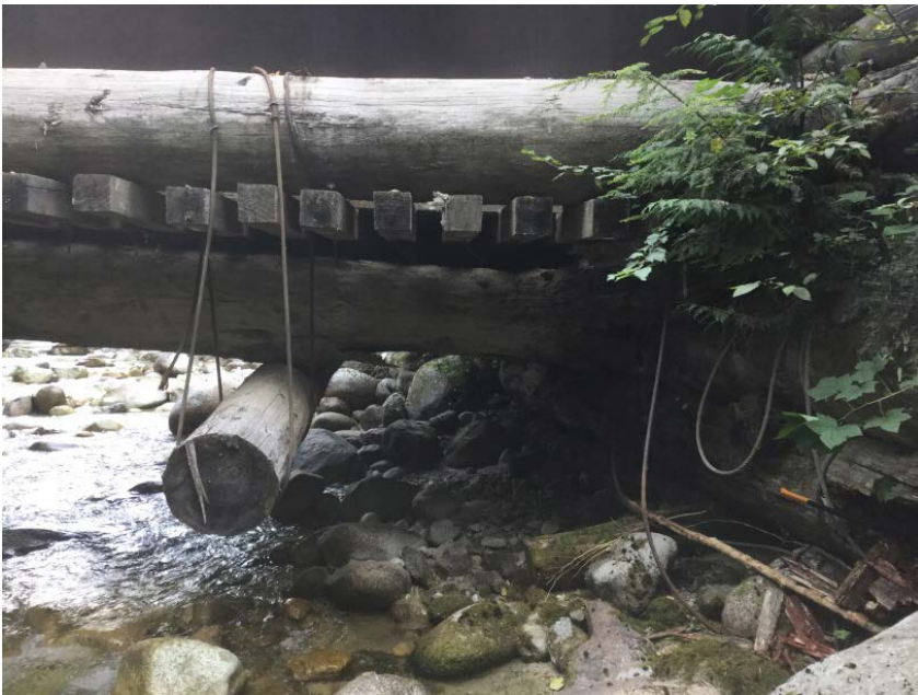
The needle beam is holding the stringer up
